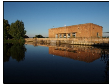
Gold Corner Pumping Station
